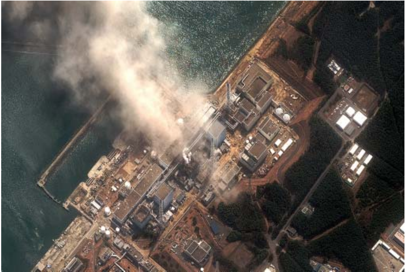
March 14, 2011: Satellite images of Japan showing damage after an Earthquake and Tsunami at Dai Ichi Power Plant, Japan. These were taken at 11 : 04am local time, 3 minutes after an explosion. ( DigitalGlobe )
